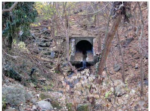
Figure 5 - Culvert Outfall
